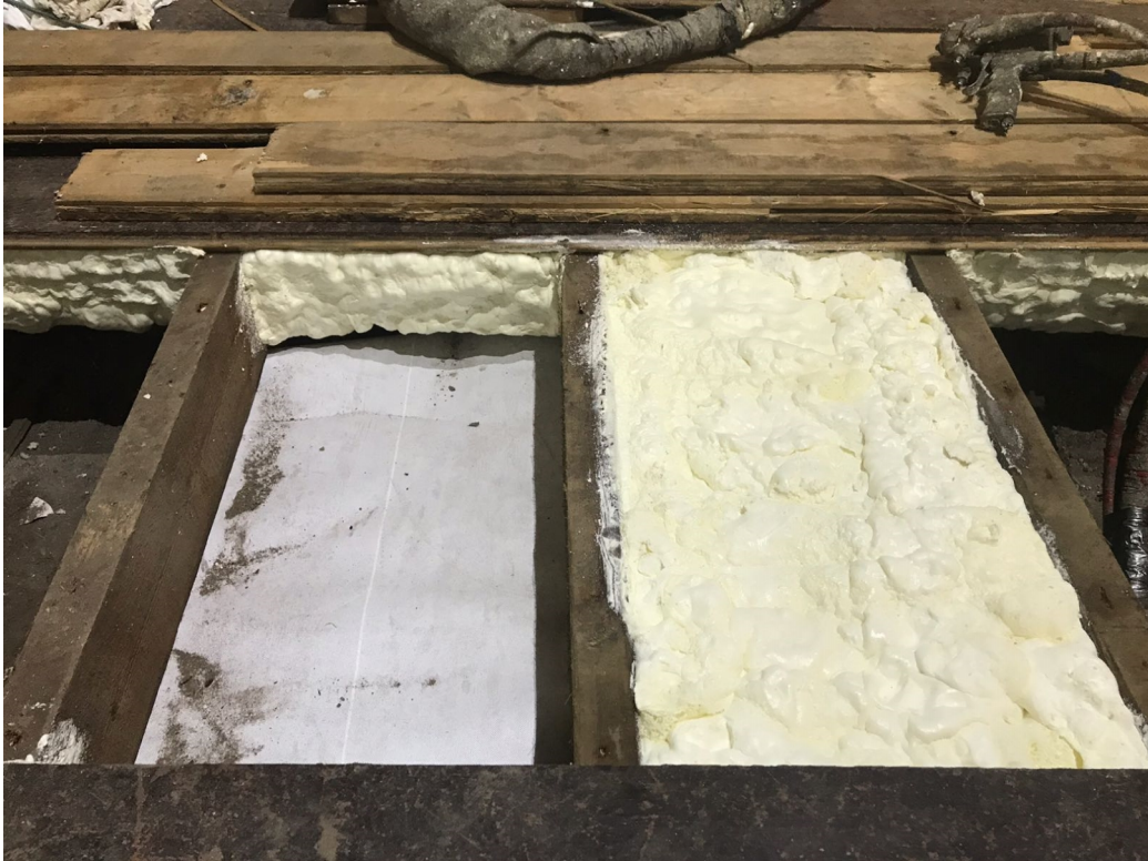
Figure 1 - the Product installed between joists - before and after
